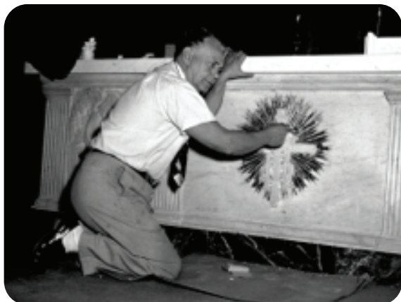
Hugo Ohlms at work on the altar of the Cathedral Basilica
